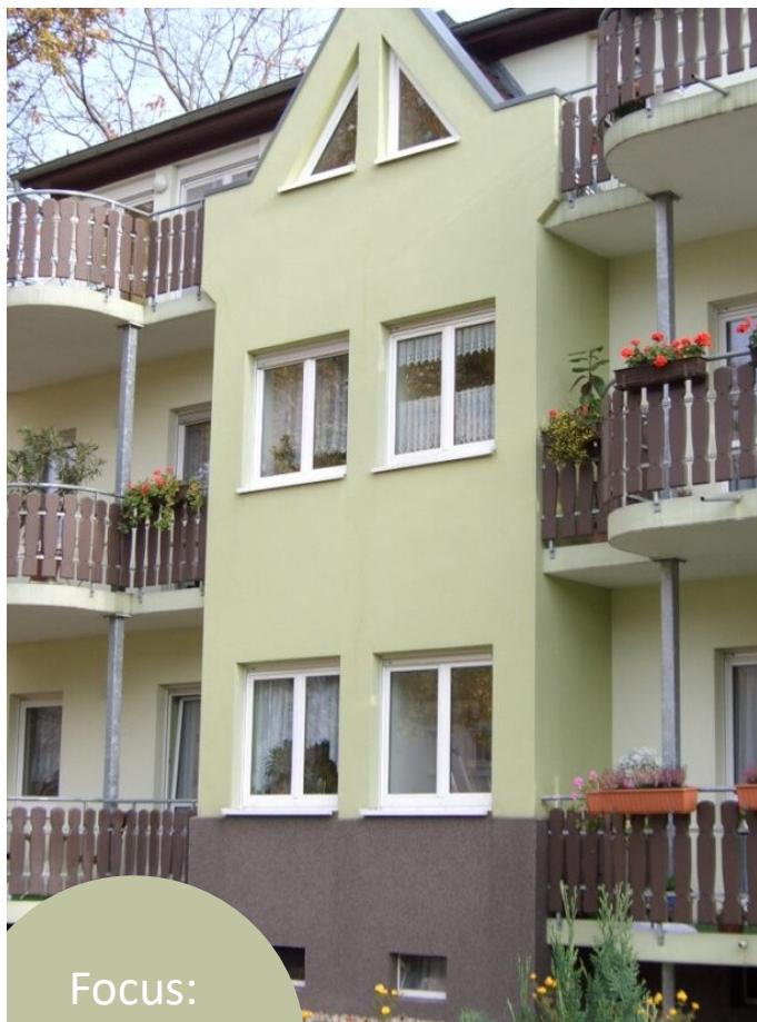
The owner of the property is a painter himself and a recognized building protection expert. At the time, he deliberately decided against additional insulation and instead opted for a climatic coating from SICC Coatings both inside and out.
