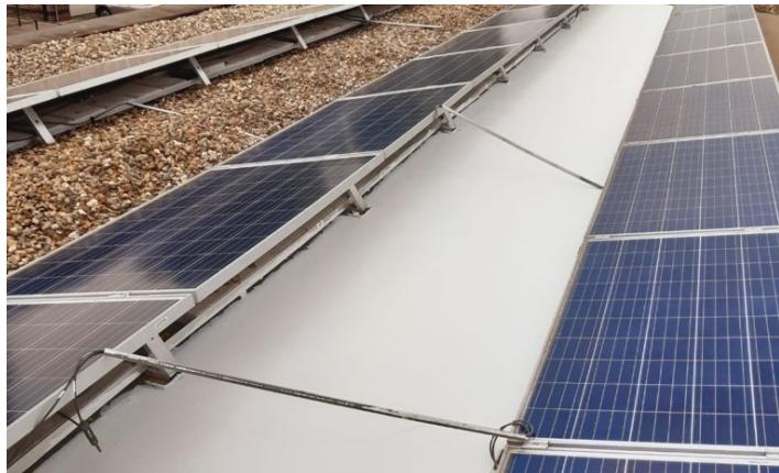
For many modules, the energy yield decreases by 0.35% for every degree Celsius increase in temperature. That doesn't sound like much at first, but with a temperature difference of 10°C, that is already 3.5% less energy generated.
